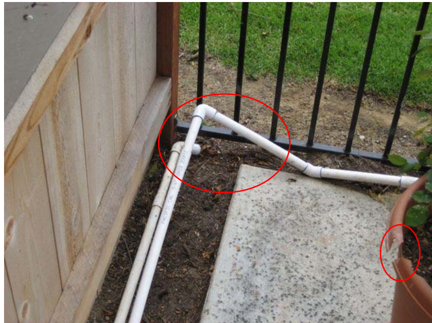
Picture Eight – Cracked Pot and unearthed pipes
